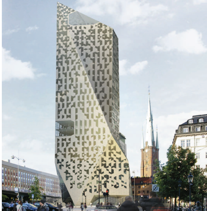
Figura 6.13. Continental Tower Block
