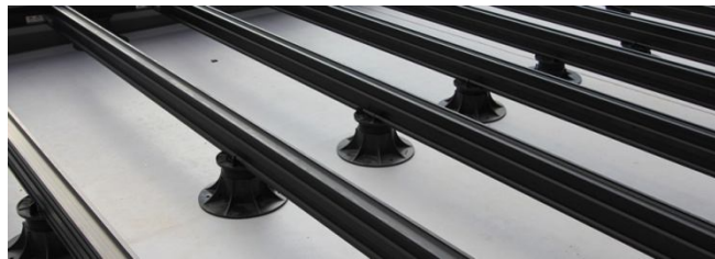
Figures 4.41, 4.42, 4.43 decking system of the wooden pavement of the new parts
