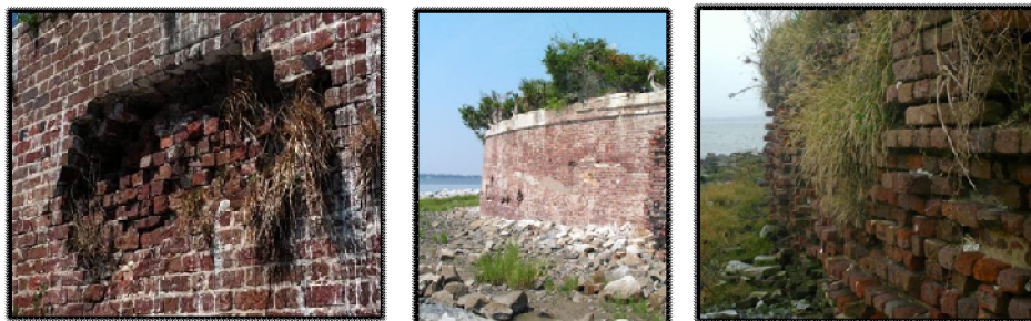
Figures 4.11, 4.12, 4.13, missing bricks of the outer layer of the walls
