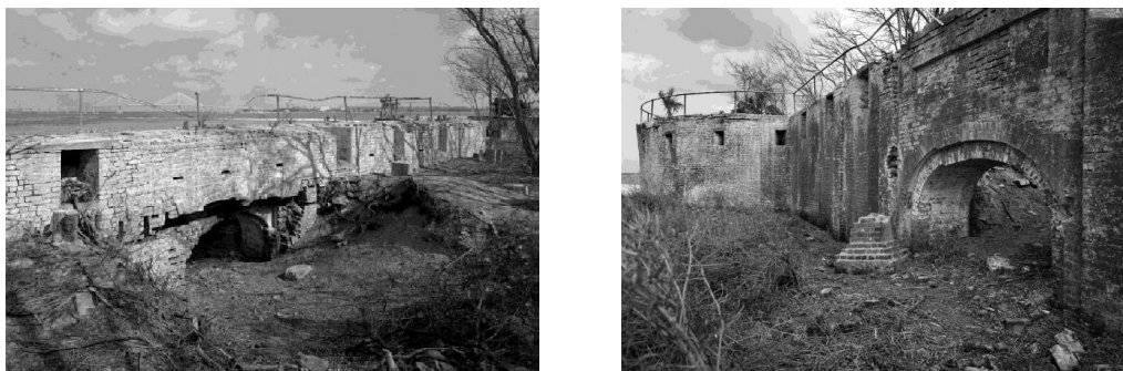
Figures 4.28, 4.29, poor condition of the joints and mortar in Castle Pinckney
