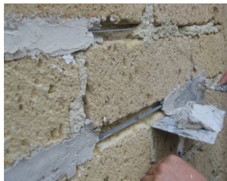
Figure 4.30, near-surface reinforcement of the walls
