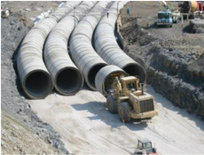
Figura 2.2: condotte idriche in calcestruzzo armato. "Federal Highway Administration", US Department Of Transportation
