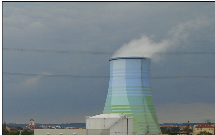
Figure 1.1 Example of a DCHX: in a cooling tower, the warm liquid mixes with ambient air. A portion of the water brings the air to saturation, and the rest goes in a container at the bottom of the cooling tower (cooling tower in Dresden, Germany)
