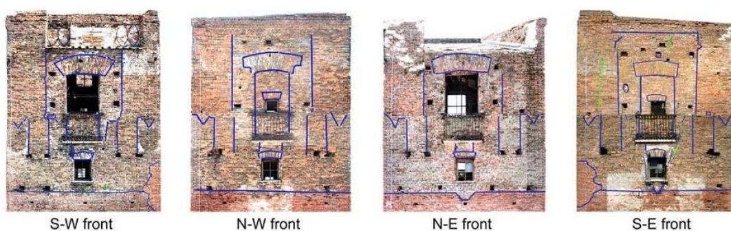
Figure 0-3 Map of the discontinuities on top of the "Gabbia" tower.
