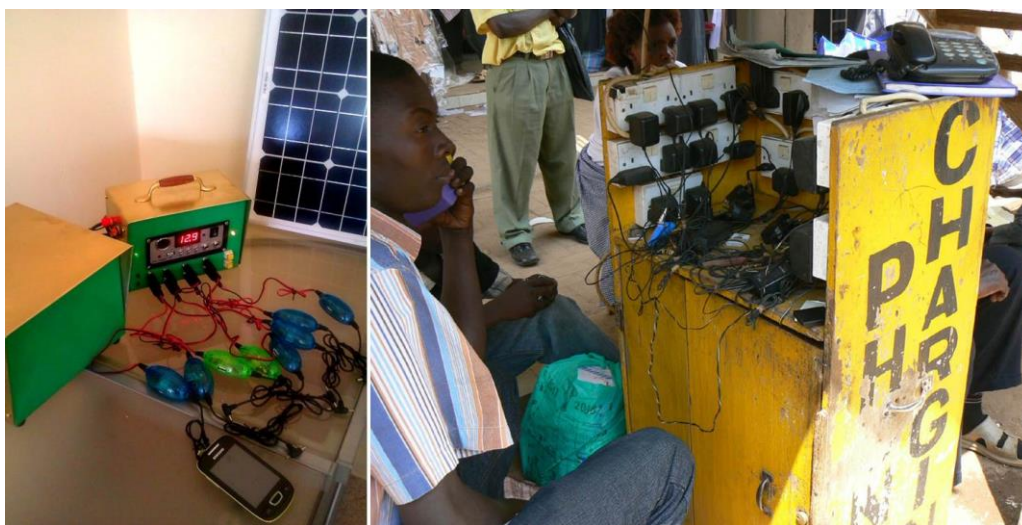
Fig 1.13 Village Energy phone charging system on the left and a typical phone charging business in rural context on the right.
