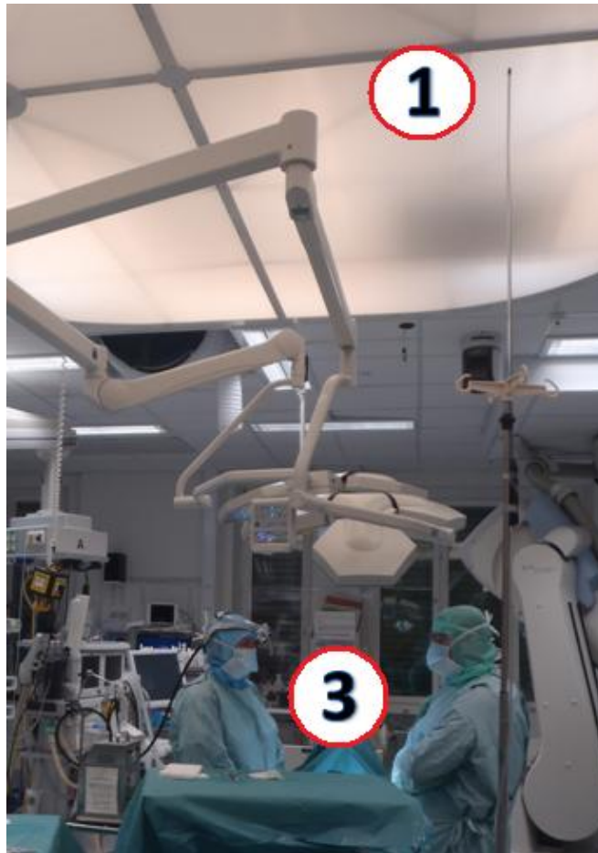
Figure 5.7. The two instrument positions defined for the measurements performed during the simulated surgery (operation N°22). Position 1 indicates the sampling probe position of UPC that measures the UFP under H14 HEPA filters. In position 3 the UPC and OPC were placed to detect the airborne particle concentrations close to the surgeon's nose.
