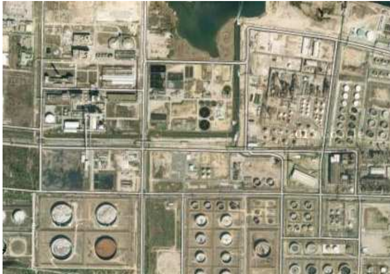
(a) Real map of the zone used for the first set of tests (the building must not be considered and water is not deep)
