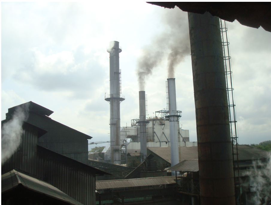
Chimneys of the boilers. Boiler 7 (highest chimney) is provided by electro-filter
