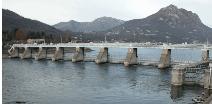
Figure 2.1: View of the Olginate dam
