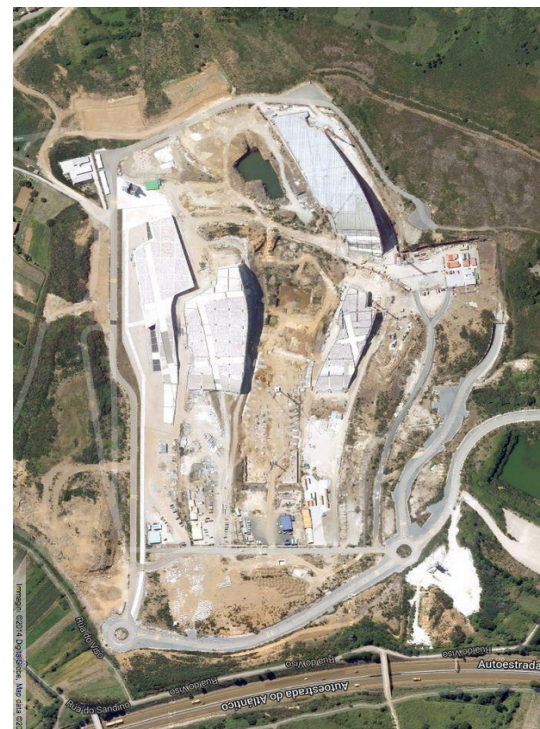
L_ Costruction site
