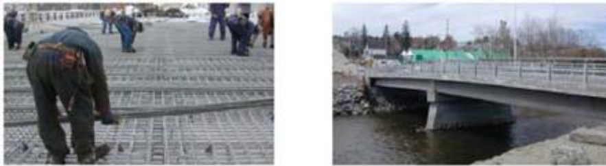
Figure 12: Bars in a bridge
