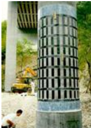
Figure 11: Example of column wrapped to increase the bearing capacity
