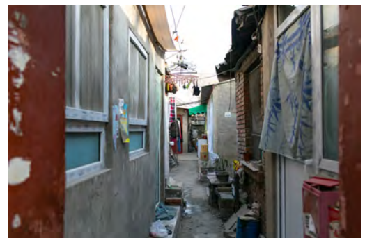
52. a dilapidated courtyard, photo credits: http://2.bp.blogspot.com/
