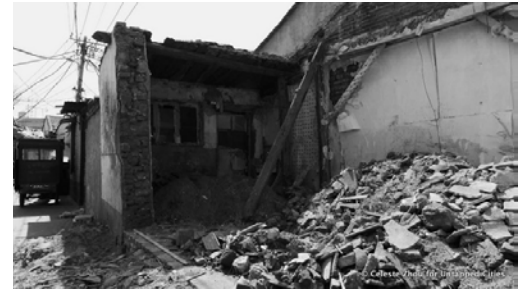
45. a demolished siheyuan, photo credits: http://untappedcities.com/
