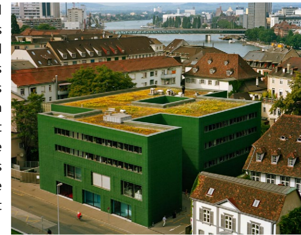
fig3.4.1 The rossetti building of cantonal building green roof
