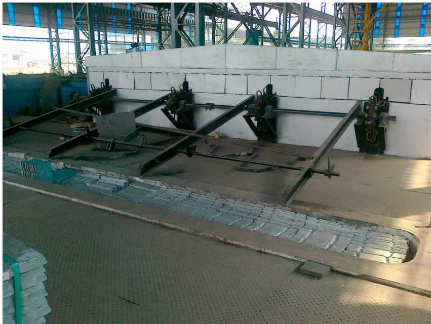
Figure 1-6 Retrofitted zinc pot and pre-heater exit. Courtesy of DCHP
