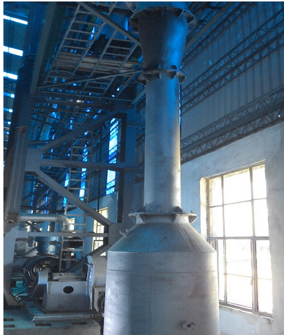
Figure 1-7 Ejector-stack. Courtesy of DCHP
