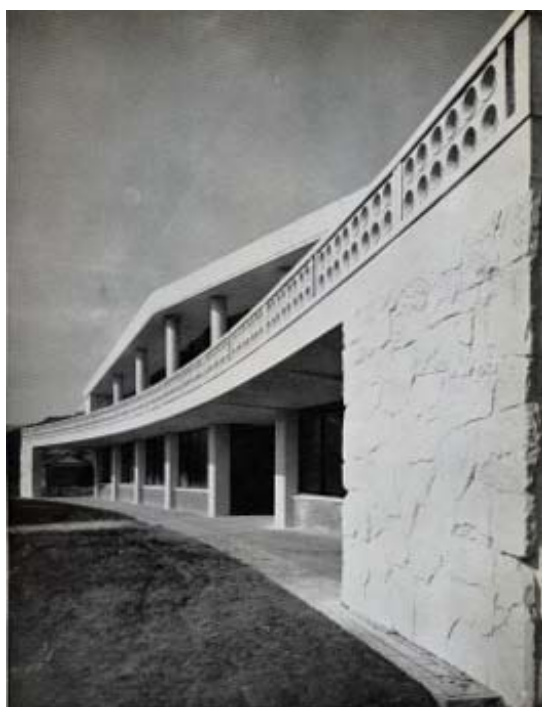
figure 1.7: Matsuidamachi city hall
