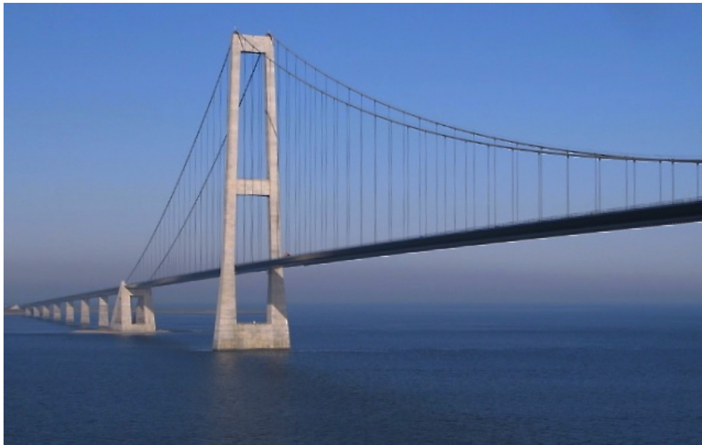
Figura 1: Storebaelt East Bridge - Danimarca (foto: Theomin - Flickr 2008)
