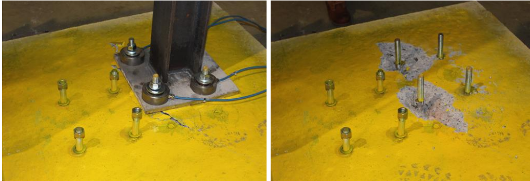
Figure 5.17. Failure mode of the post HEA120.
