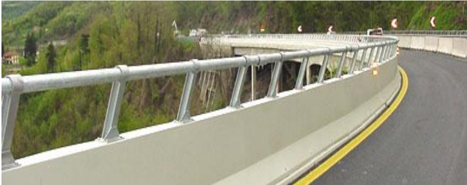
Figure 6.2. Example of concrete barrier.
