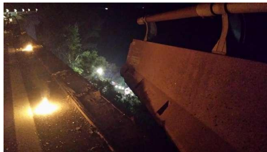
Figure 1.4. Example of accident involving bridge safety barriers (Avellino, July 28 th 2013) [5].
