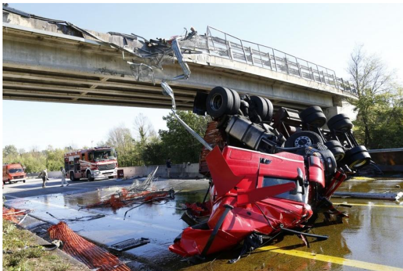
Figure 1.1. Example of accident involving bridge safety barriers (Siena, October 13 th 2013) [3].
