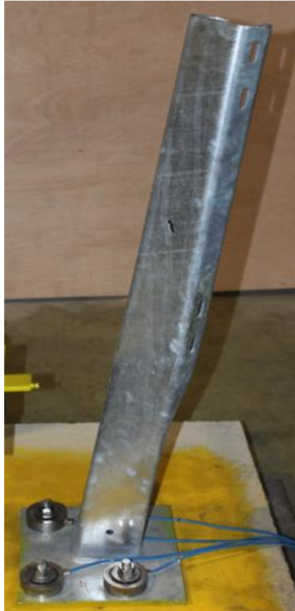
Figure 5.9. Failure mode of the post C125.
