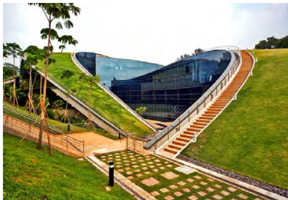
Figure 3-32 Access to the Green Roof, Nanyang Technical University, Singapore
