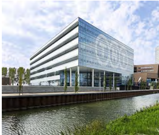
Figure 3-28- External View - TNT Head Office, Netherland
