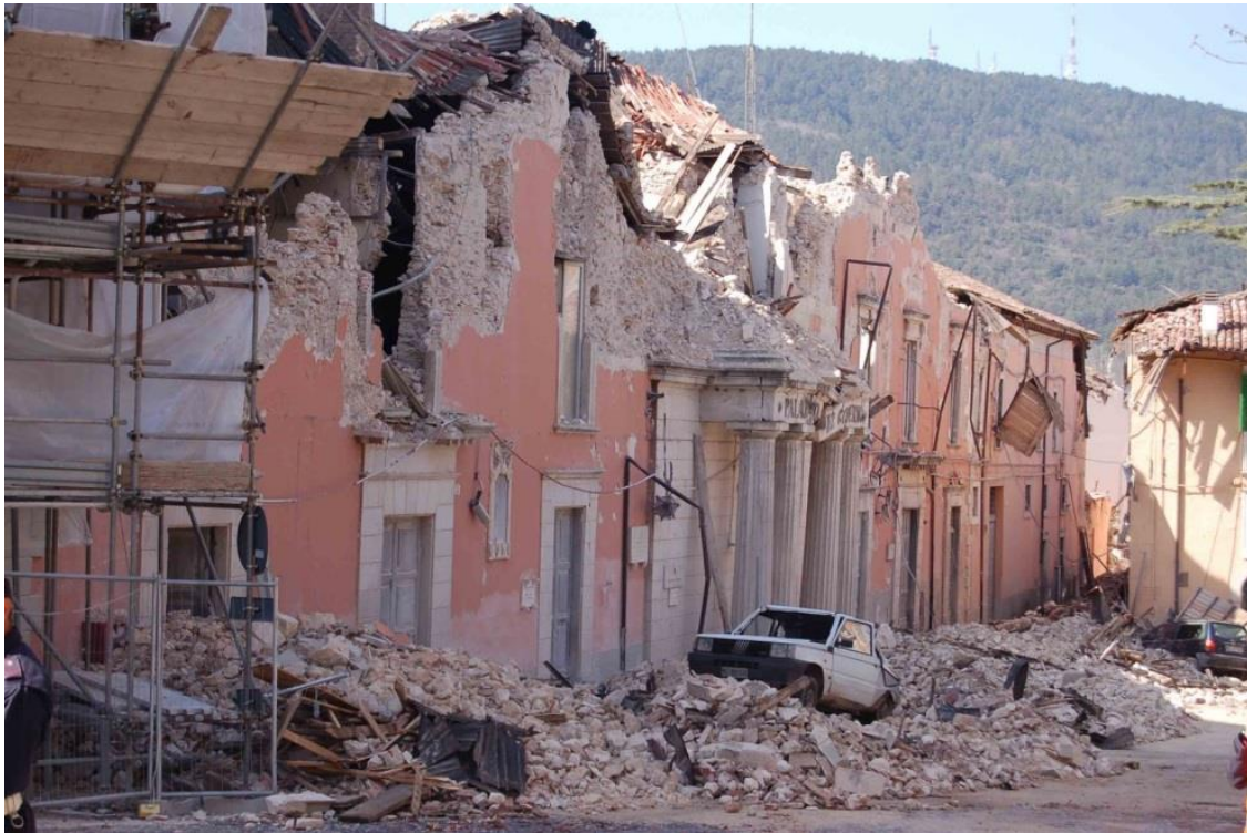
Figure 1-2: L'Aquila after the earthquake of 2009, April 6. Magnitude 5.8, Mercalli IX
