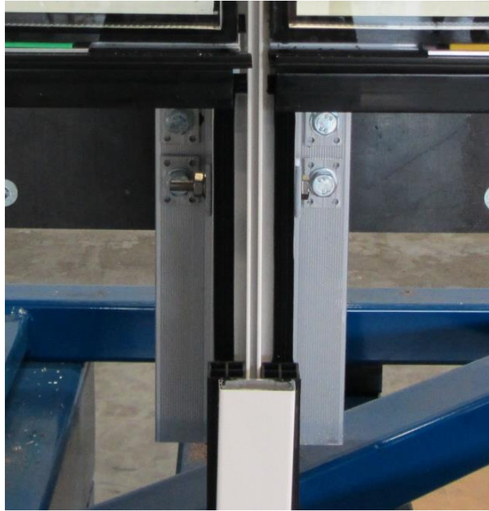
Figure 8-13: : picture of a fixed anchor
