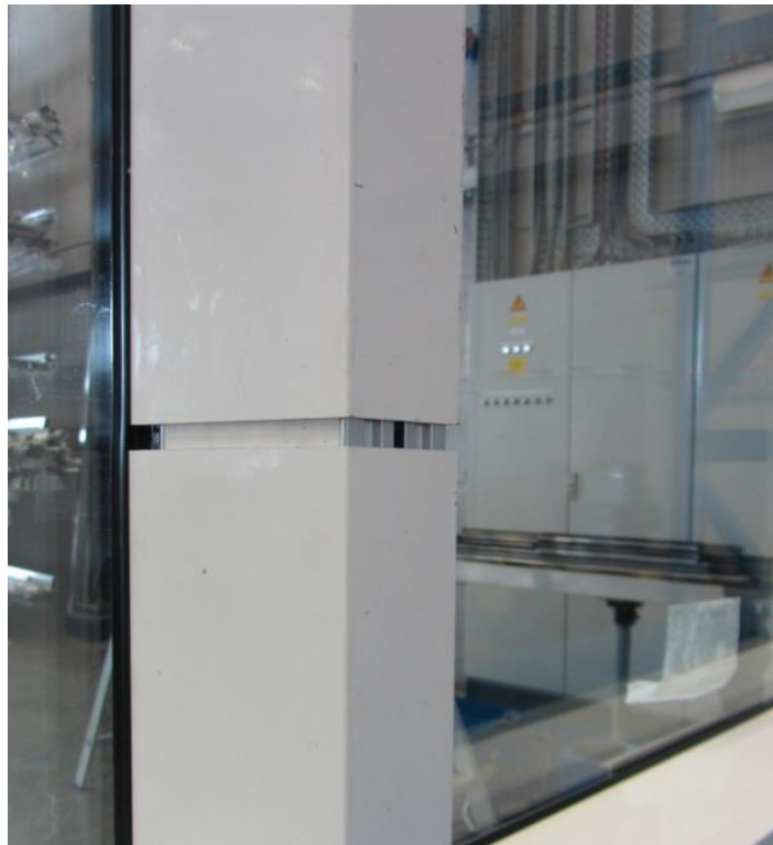
Figure 8-14: : picture of a dilatation joint
