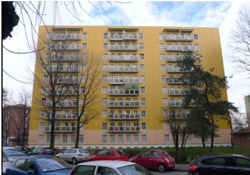
Fig 6. 5: the building after
