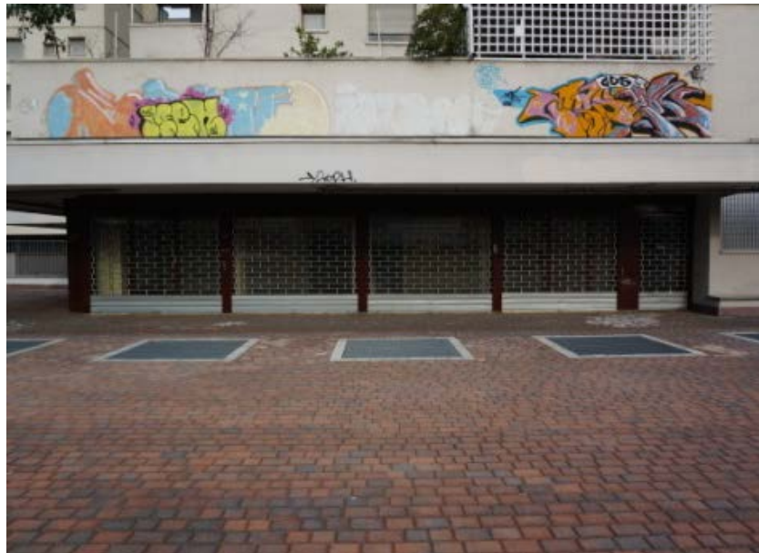
Fig 6. 6: the empty ground floor of the tower (photo taken by author)
