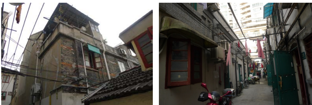
Fig 7. 13: the house inside the neighbourhood after the regeneration (photo taken by author)
