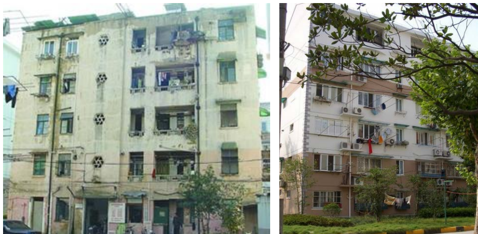
Fig 7. 6: the building before and after the regeneration 13
