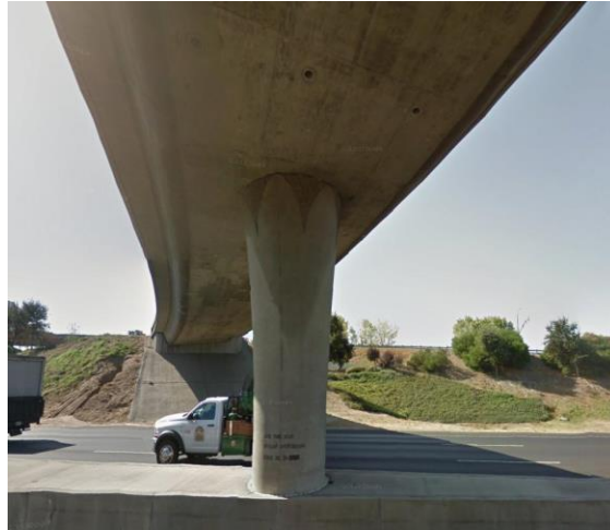
Fig. 3.2. Single pier of the Bridge A.
