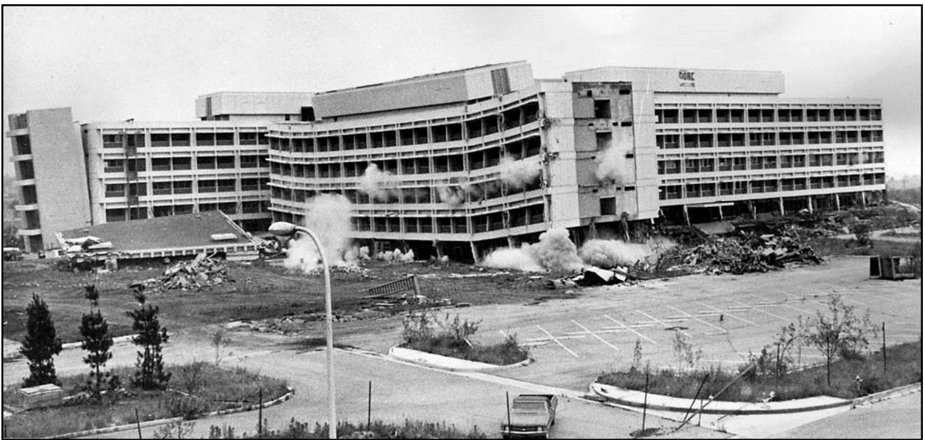
Figura 45 Sylmar Olive View hospital
