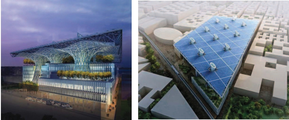
Immagine 18_Masdar Headquarters, Abu Dhabi
