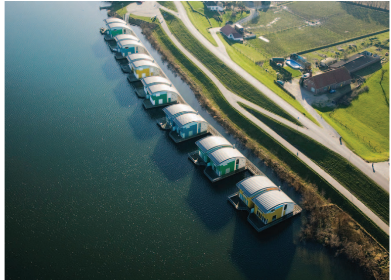
FIG. 4.4.3 Floating dwellings in Maasbommel development
