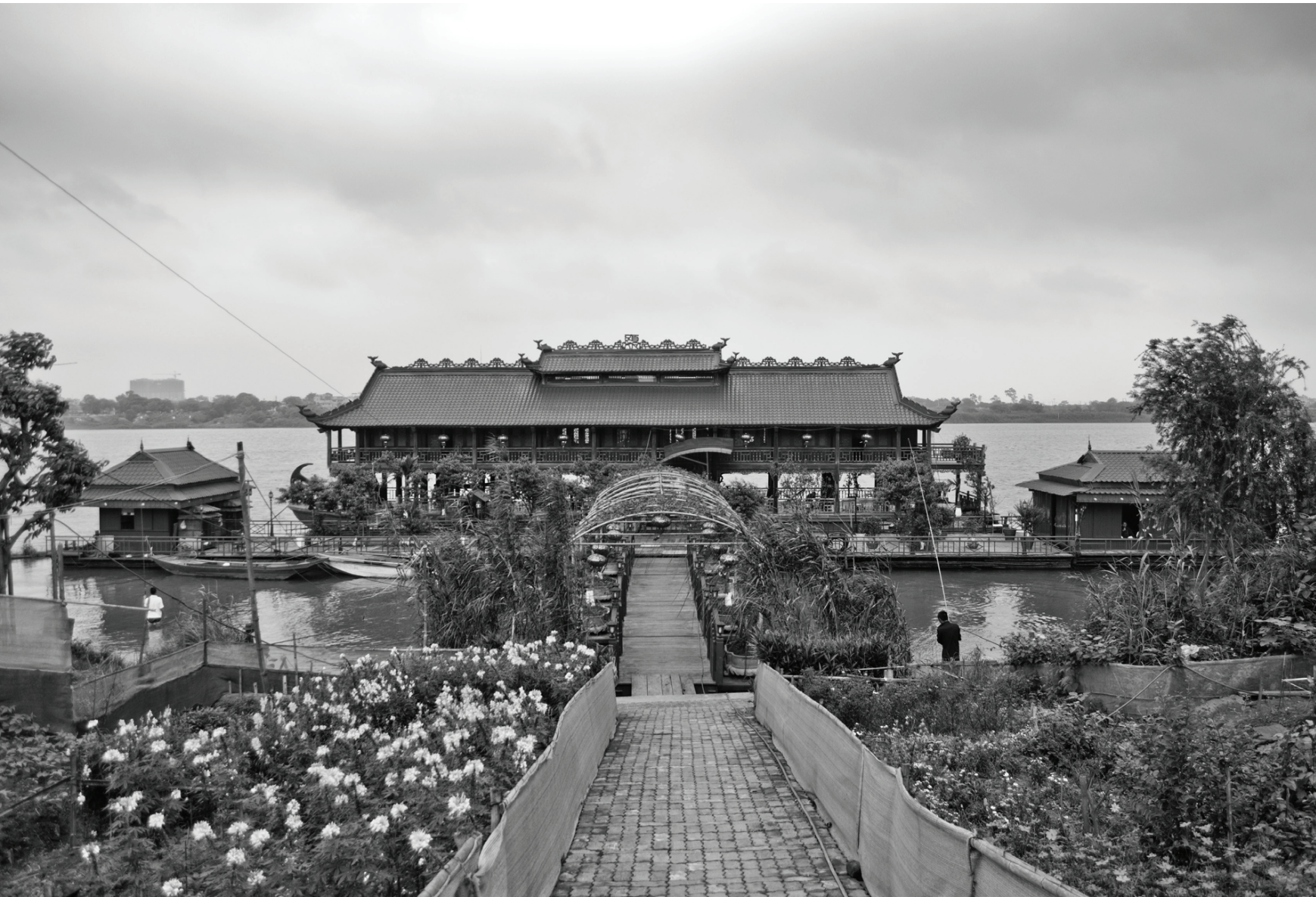
FIG. 3.3.8 Single family floating house in Chuong Duong ward. The family moved to live on the river in search for less pollution and noise from the city and to be closer to nature. Has the legal right to be there according to the owners who have been living there for 10 years now. Location Chuong Duong ward, April 2014
