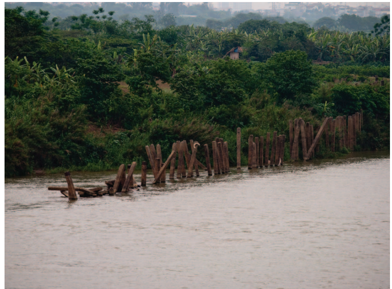
FIG. 4.1.9 Concrete pillars breaking the water flow Location: Island in the Red river, Long Bien ward, April 2014
