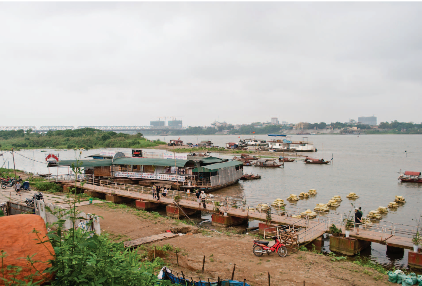
FIG. 3.7.15 Phuc Tan port. Floating pontoon staying on ground during dry season still providing access to the floating structures. Location: Chuong Duong ward, April 2014
