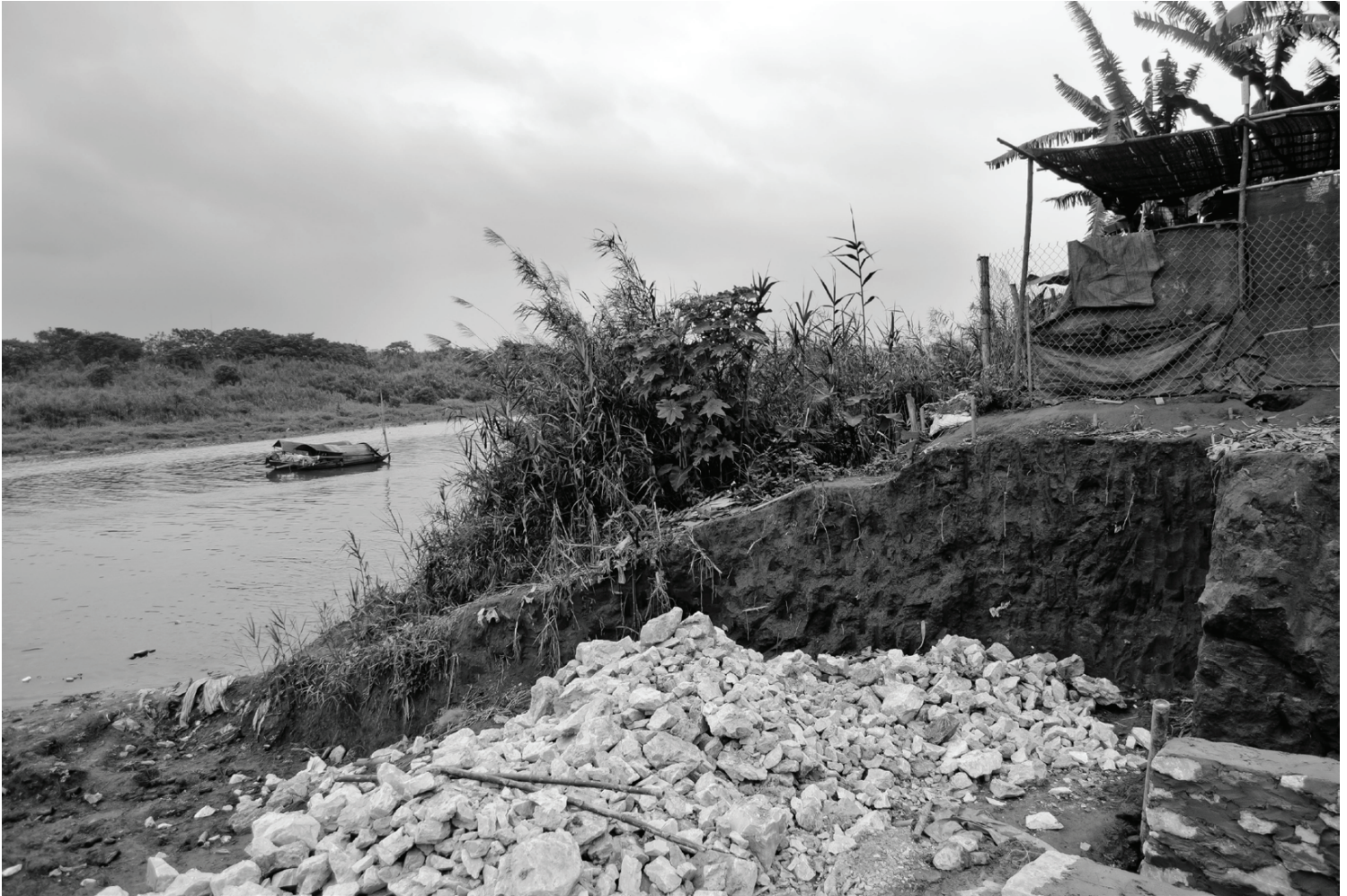
FIG. 3.5.1 River banks and dyke edge destruction due to undefined constructions. Location: Phuc Xa ward, Red rived edge, April 2014
