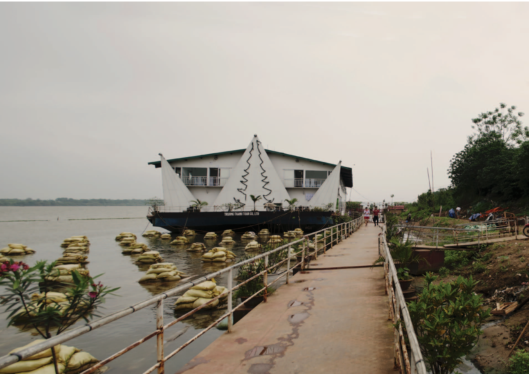
FIG. 3.7.6 High Quality floating house part of the Phuc Tan port in Chuong Duon ward during dry season. Access is provided by adapted to float metal path which at this period is partially sitting on dry ground;
