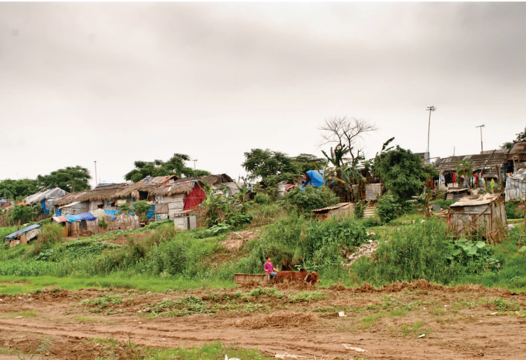
FIG. 3.7.10 Squatting in the lower lying areas in the flood plain of the Red river. Self constructed houses whose inhabitants are mainly cultivating the available land of the floodplain. Located at the foot of the step dyke they are threateting the safety of the dyke Location: Tu Lien ward, April 2014
