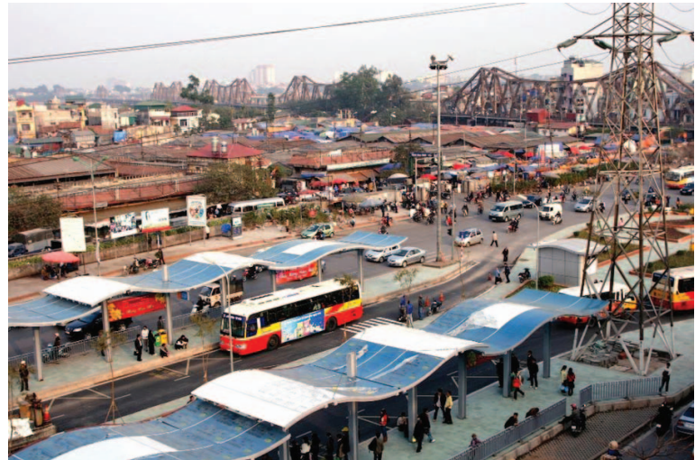
FIG. 4.1.5 Major interchange station Long Bien, background view of the bridge and market, Source: IMV- Hanoi
