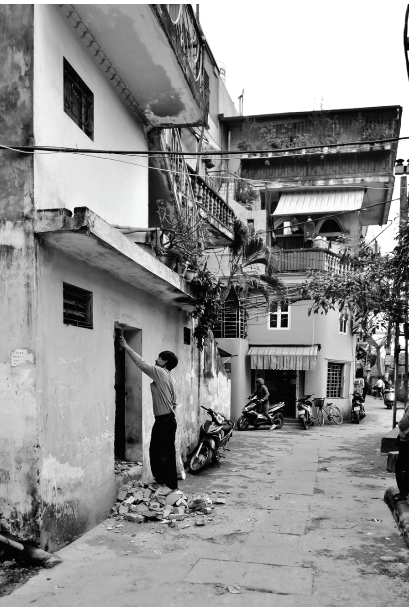
FIG. 4.5.5 Slightly elevated door in case of a flood. Location: Phuc Tan ward, March 2014
