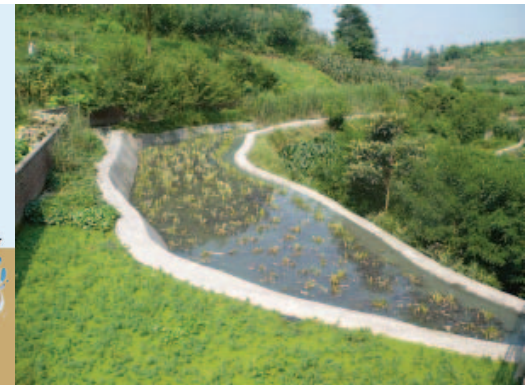
FIG. 4.5.16 Example of implemented natural purification station in Chongqing, China Source: http://elkkidsnews.wordpress.com/
