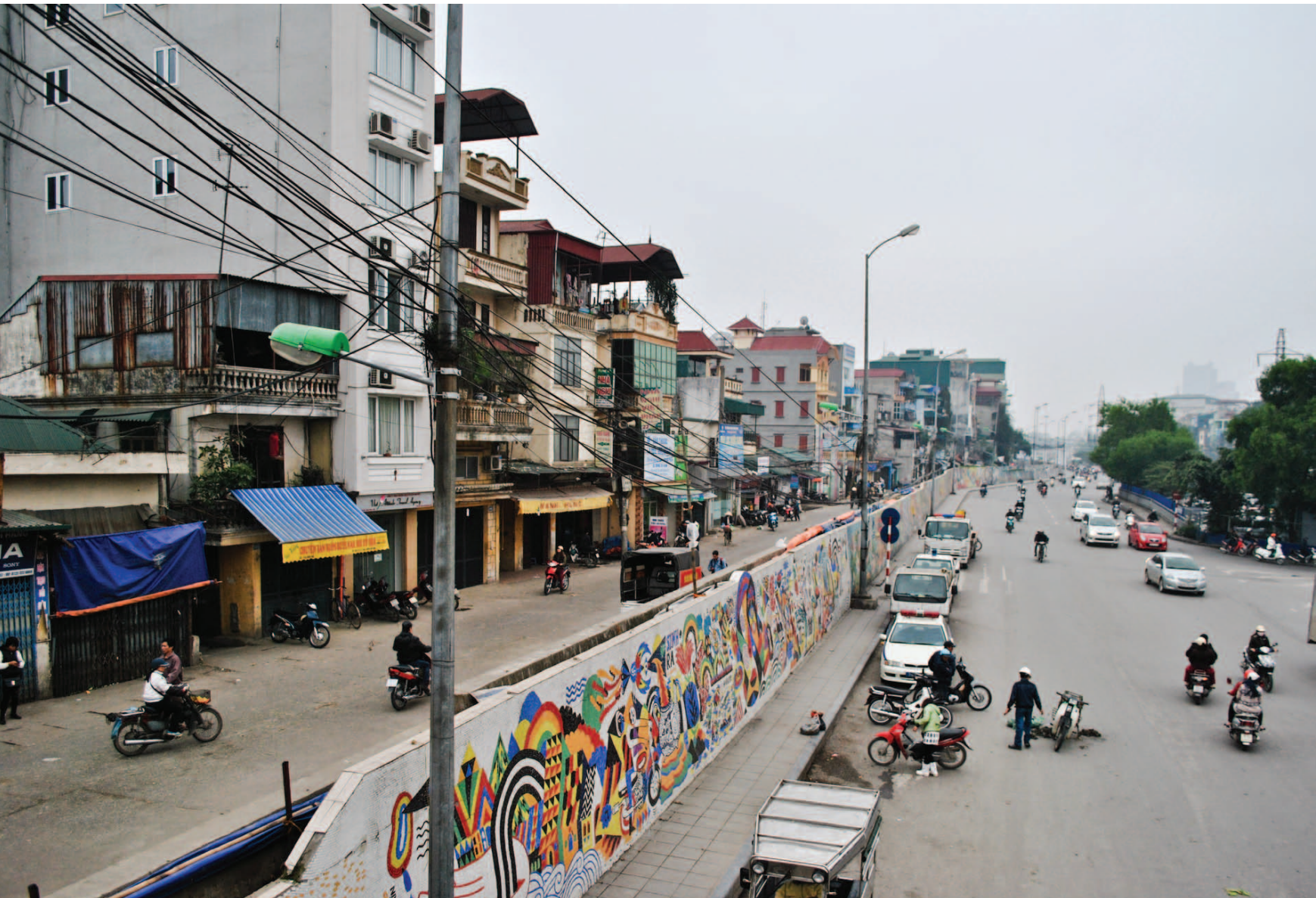
FIG. 3.7.2 The 2 meter tall dyke wall built during the 90's to increase the protection of Hanoi to floods as high as 15m is separating the historical center of Hanoi from the Riverside Urban Areas Location: Long Bien bridge, Phuc Tan ward, March 2014
