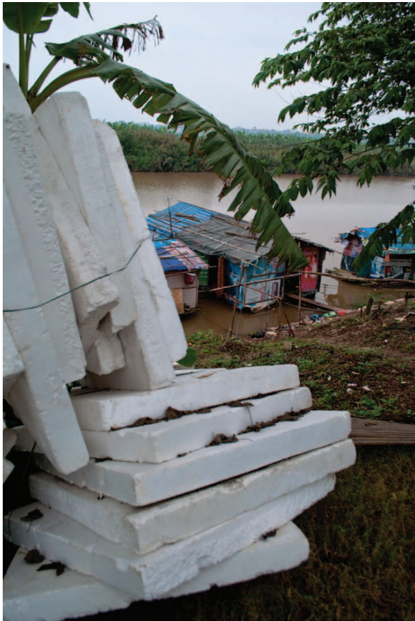
FIG. 4.4.8 Polystyrene to make the base for the floating structure. Background a floating house in Nha Van Hoa, on the island (#1 on 4.4.9)
