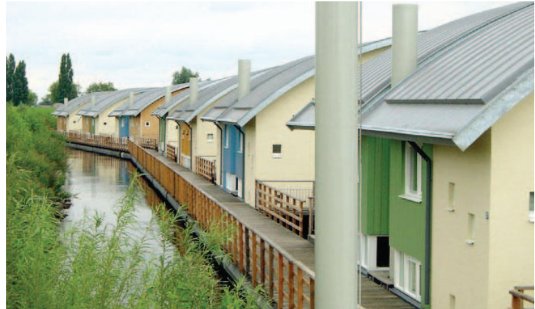
FIG. 4.4.5 Floating homes in Maasbommel, normal water level
