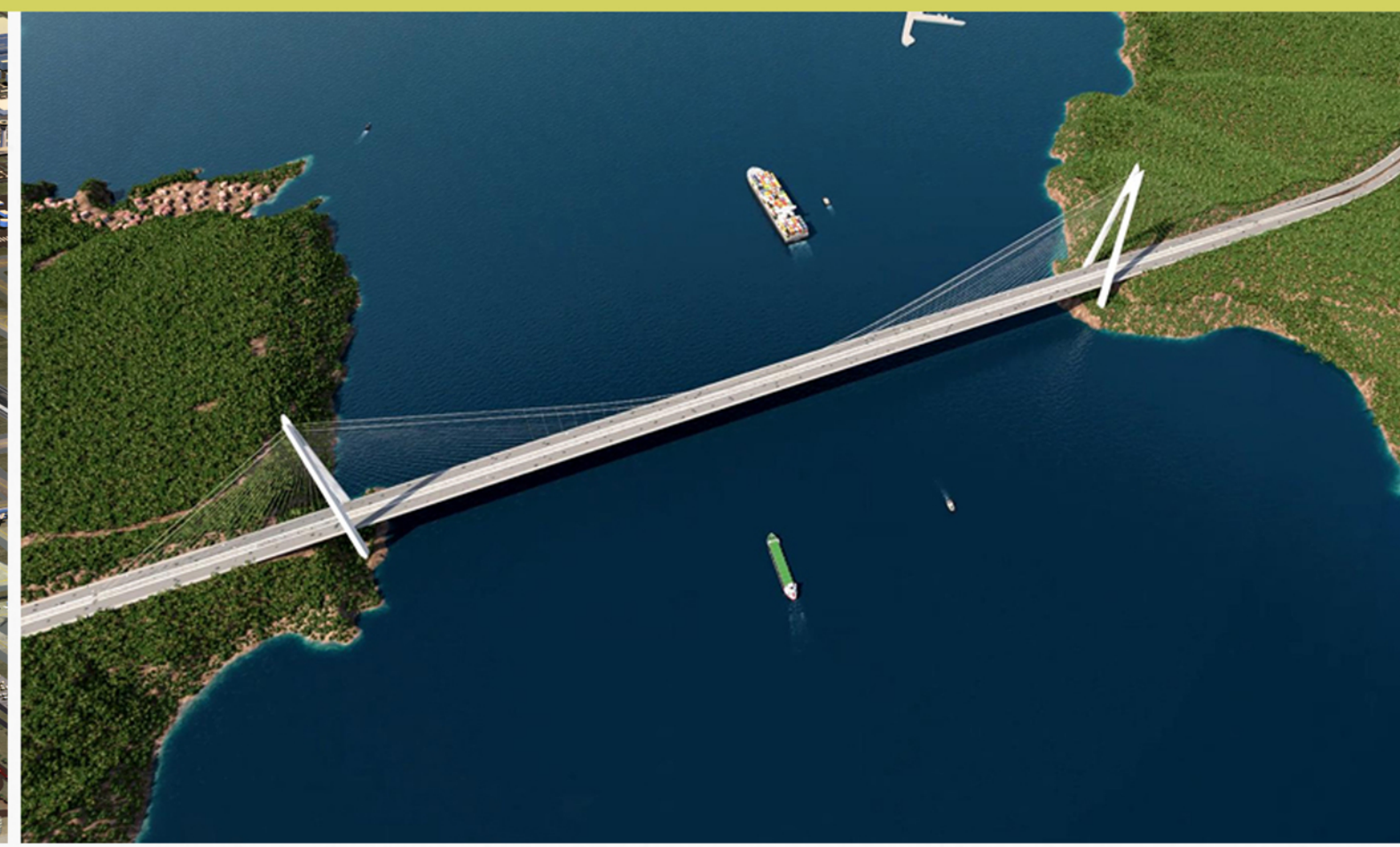
3. YAVUZ SULTAN SELİM BRIDGE
