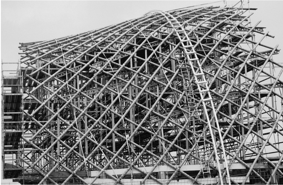
1.12 Japanese Pavilion, Hanover, Germany, by : Shigeru Ban Architects. In : Performative Architecture.
