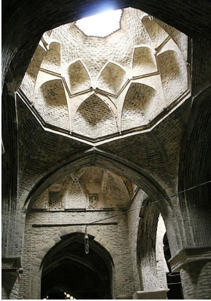
Figure 48: Patkaneh vault, Jameh mosque, Isfahan
