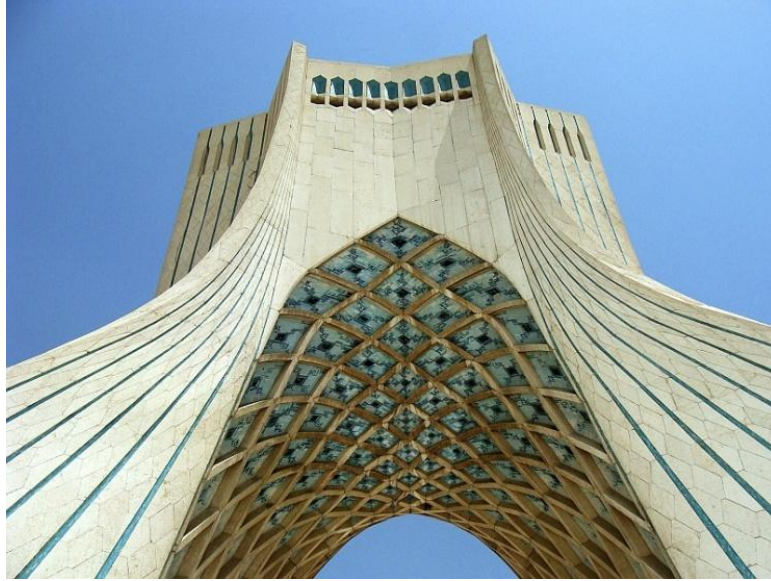
Figure 17: Shahyad tower, modern combination of ribs
