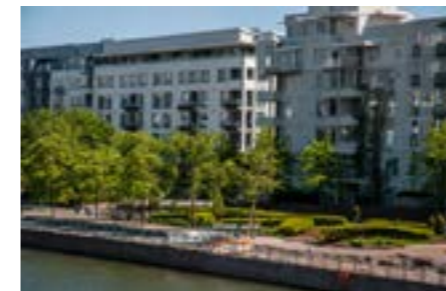
Image 5a: Ruoholahti, Finland. Apartment buildings looking at the Jaalaranta Park. Source: http://www.vihreatsyliit.fi/en/?p=921
