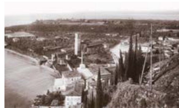
Image 35a: Toscolano around 1914. San Pietro e Paolo Church with new nearby Maffizzoli Paper mill behind and olive plantations on the Promontory. City center right. Source: (De Rossi, Fava 2003. Fondazione Negri)
