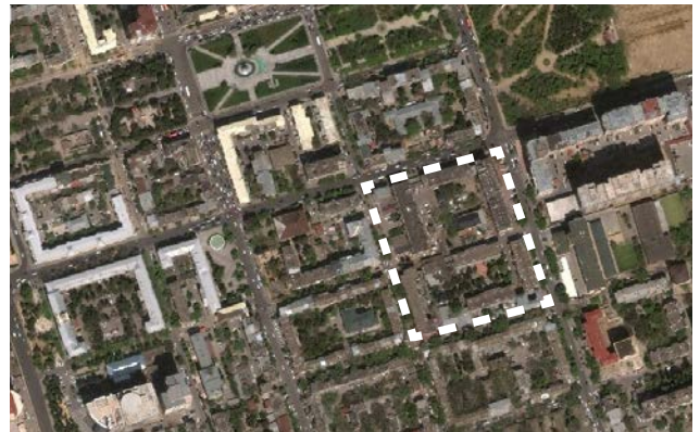
8 Azerbaijan State Oil Academy Dormitories, Bakixanov Street, 52
