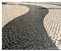
Change in pavement
