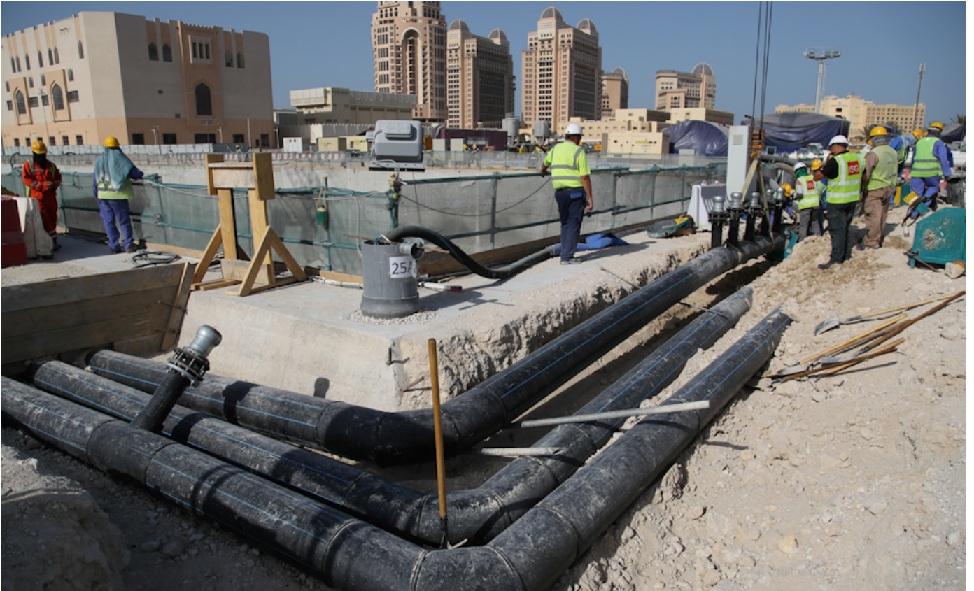
Figure 11: Installation of HDPE pipes
