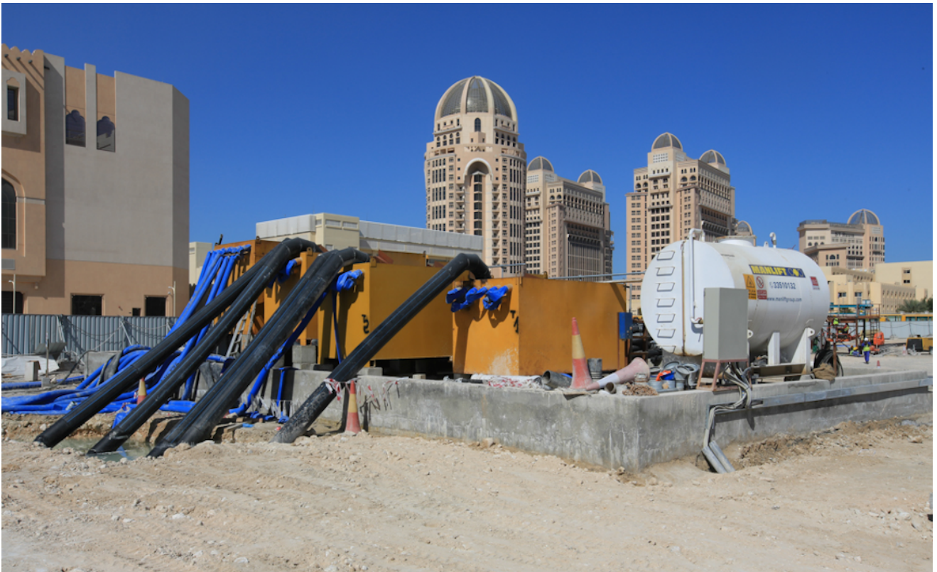
Figure 10: Replacement of Dewatering Hoses
