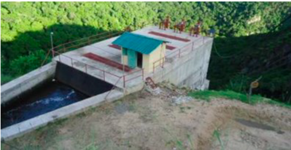
Figure 9: Hydroelectric plant on the Mpanga River
