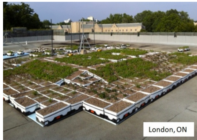
Figure 4.19: Green roof site at Western University (reproduced from [2]).
