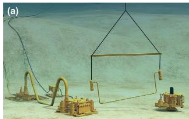
Figure 11 a & b. Vertical Tie In Jumper Installation
