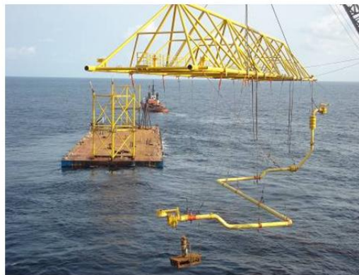
Spreader Frame for Horizontal Jumpers
