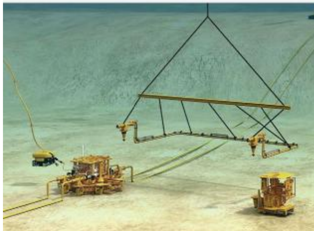
Figure 12. Horizontal Tie In Jumper
