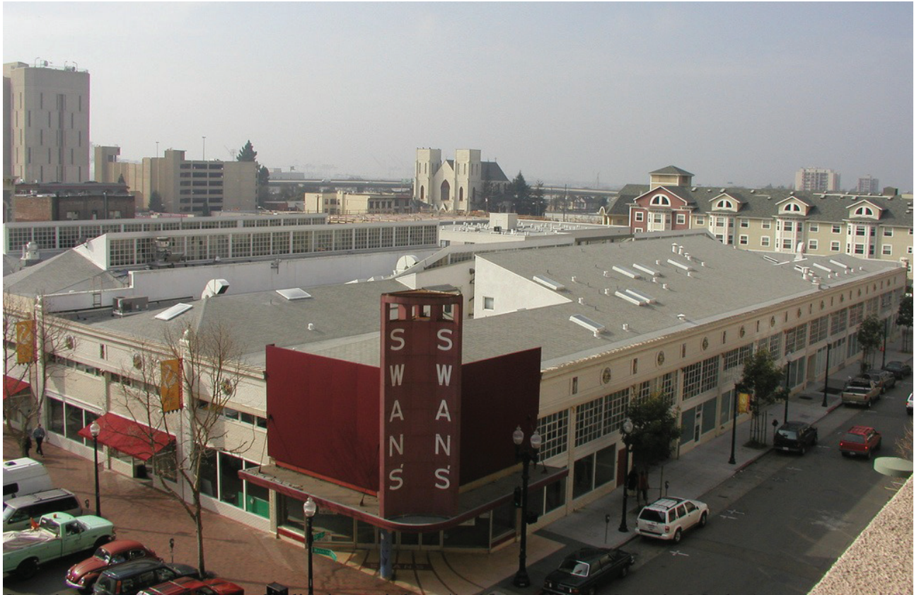
Swan's Market Co-housing, l'edificio oggi ( http://oaklandwiki.org/Swan's_Market )
