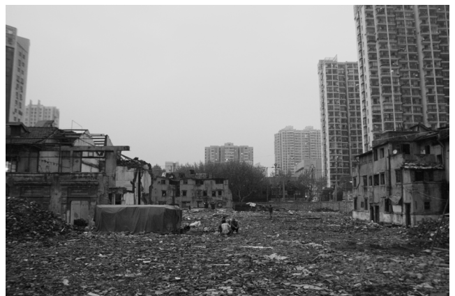
Demolished site, Tiantong road, Shanghai.
