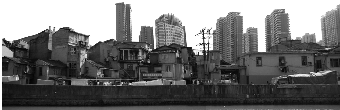
two photo-graphical reconstruction of the east side and the west side of the settlement
