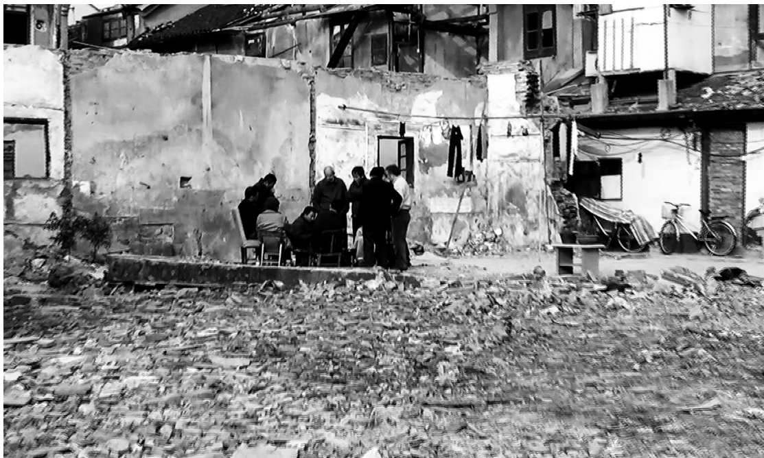
VERNACULARISM STAYS. Xingping lane demolished Lilong, Shanghai. 2014
