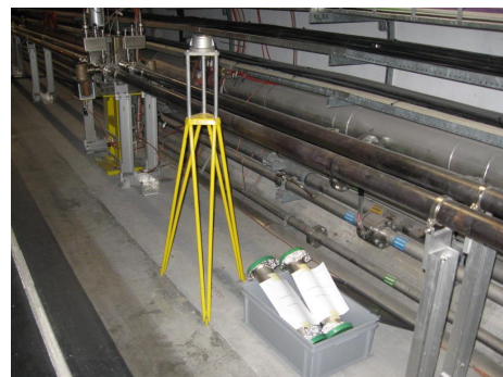
(b) Picture of the two chambers exposed in Point 3.
