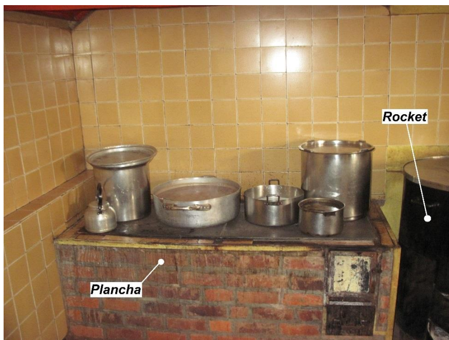
Figure 3.11 – Stoves equipment at the hospital.
