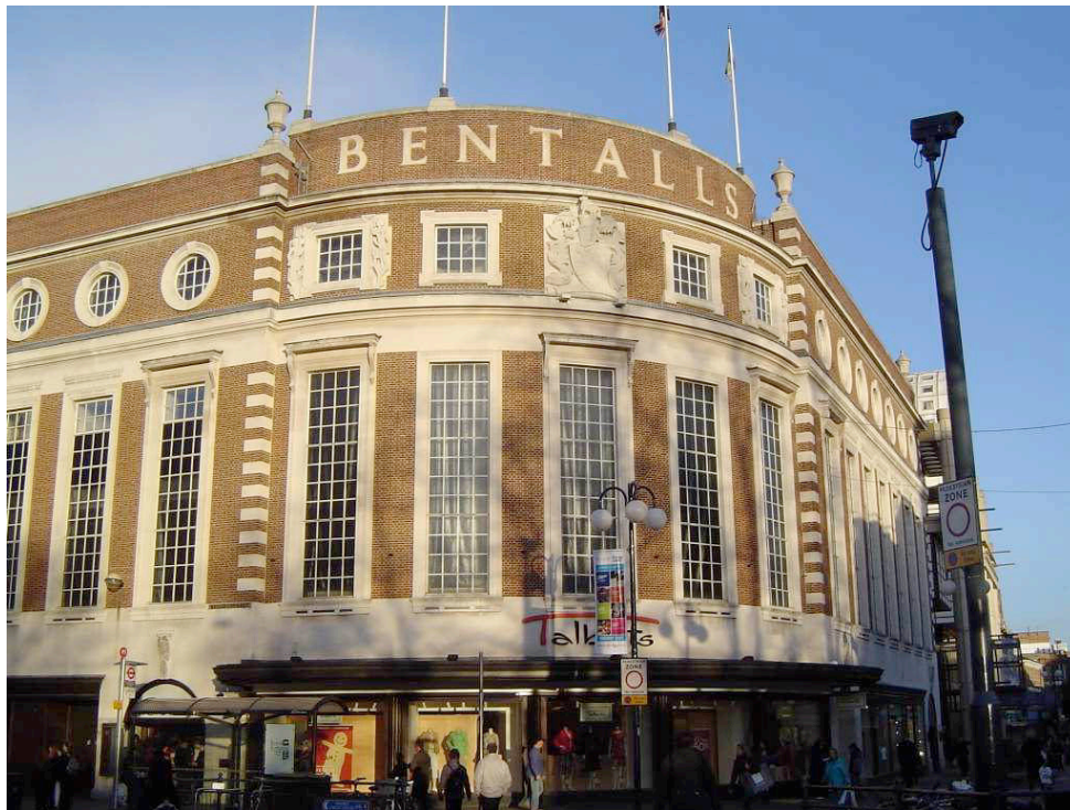
Fig. 25 Bentall's Department Store ,Wood Street/Clarence Street, Kingston upon Thames (grado II)
