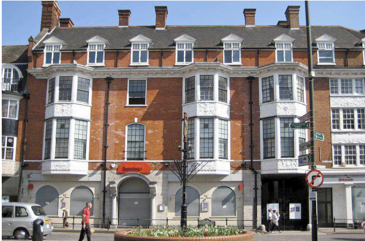
Fig. 21 Royal Bell Hotel, 173-177, High Street, Bromley, Bromley (grado II)
