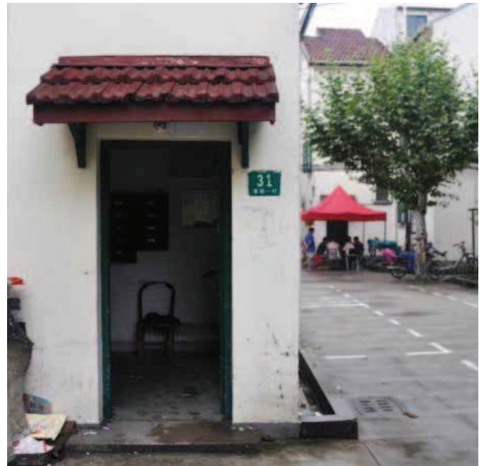
(e) Unit entrance
