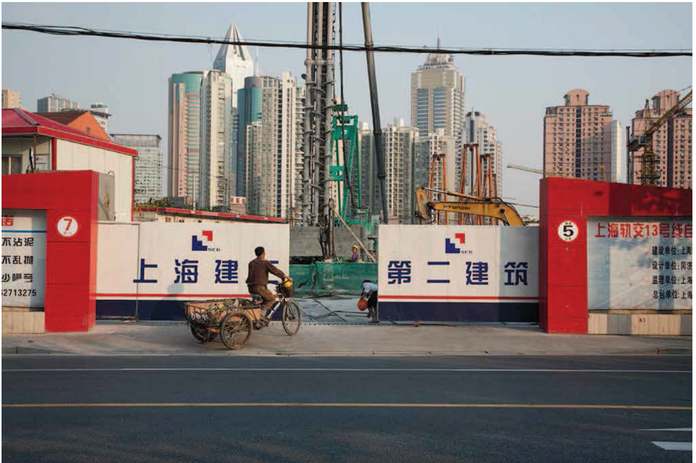
(8. 6) Shanghai Construction Group: construction site
