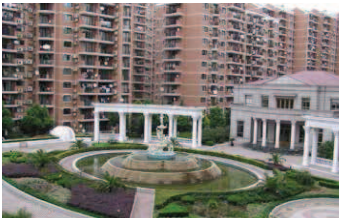
(e) Unit entrance
