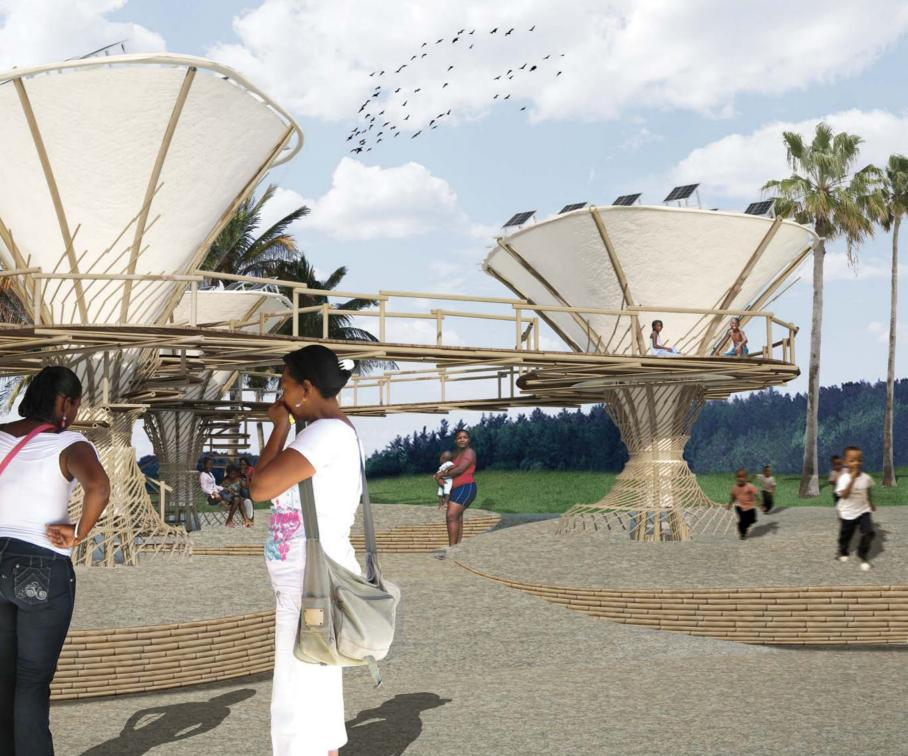
during the night, due to the high humidity; this will increase even more the water collection. Afterwards collected, the rainwater and the humidity drops will be stored in the same tank of the performed tubes of the paths, placed underground the public space.
