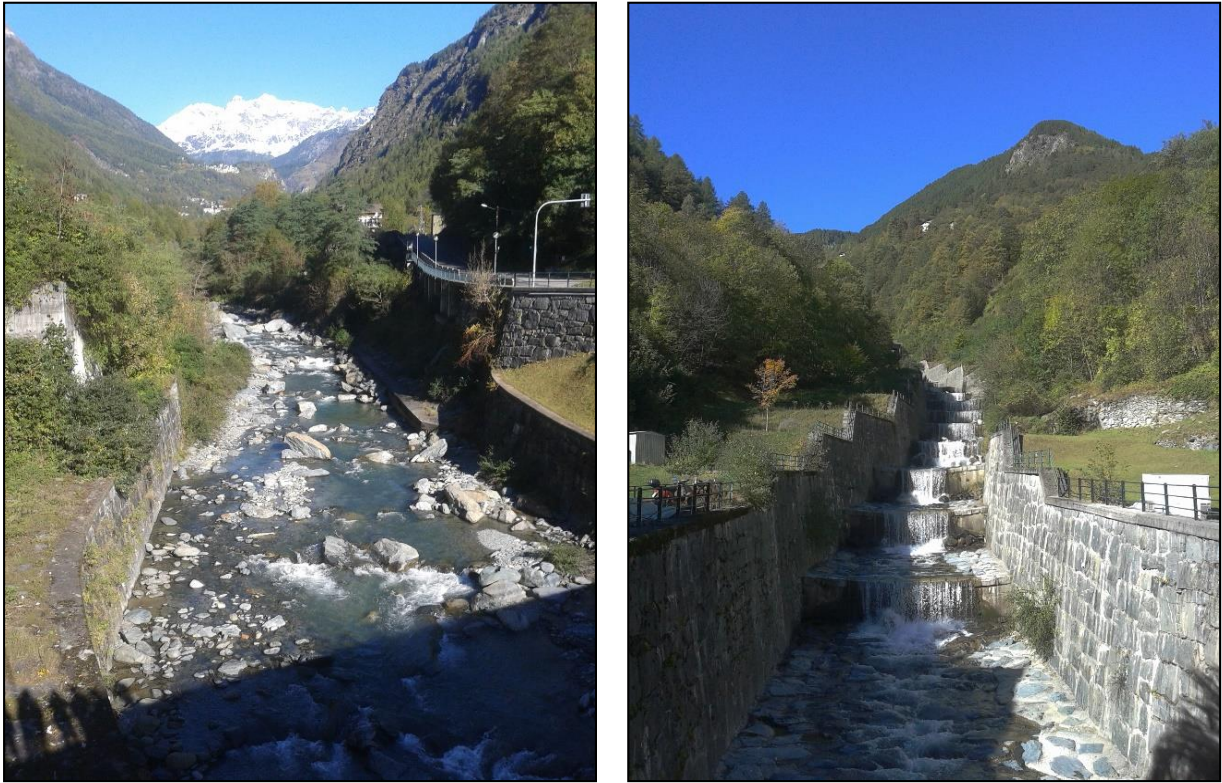
Figure I-9 Left - Mallero river near Torre di S. Maria. Right – weirs built to control the sediment yield (taken in October 2013)
