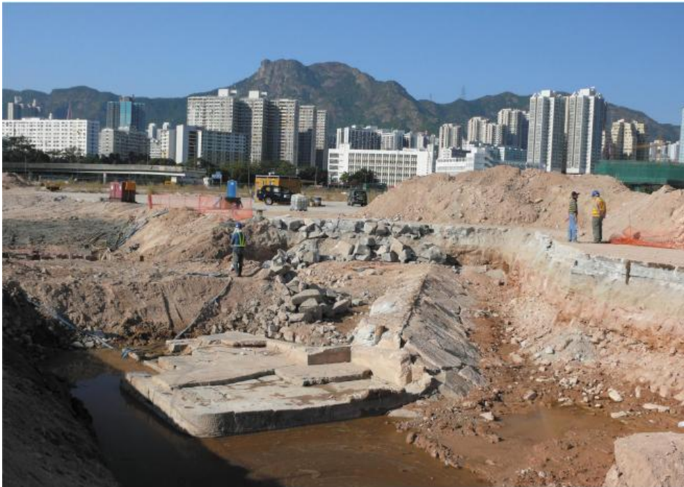
Figure 2-30 Photo of Excavation site, 2009
