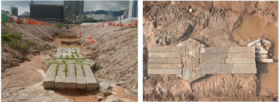
Figure 2-42 Photos of Decking on SP12 and SP13
