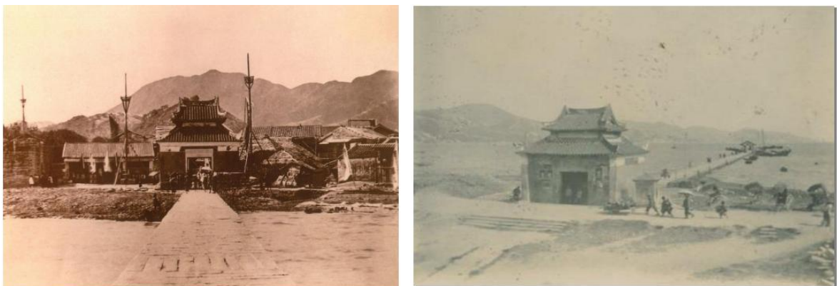
Figure 2-23 Pavilion for Greeting Officials in 1898 (left), in 1910s (right)
