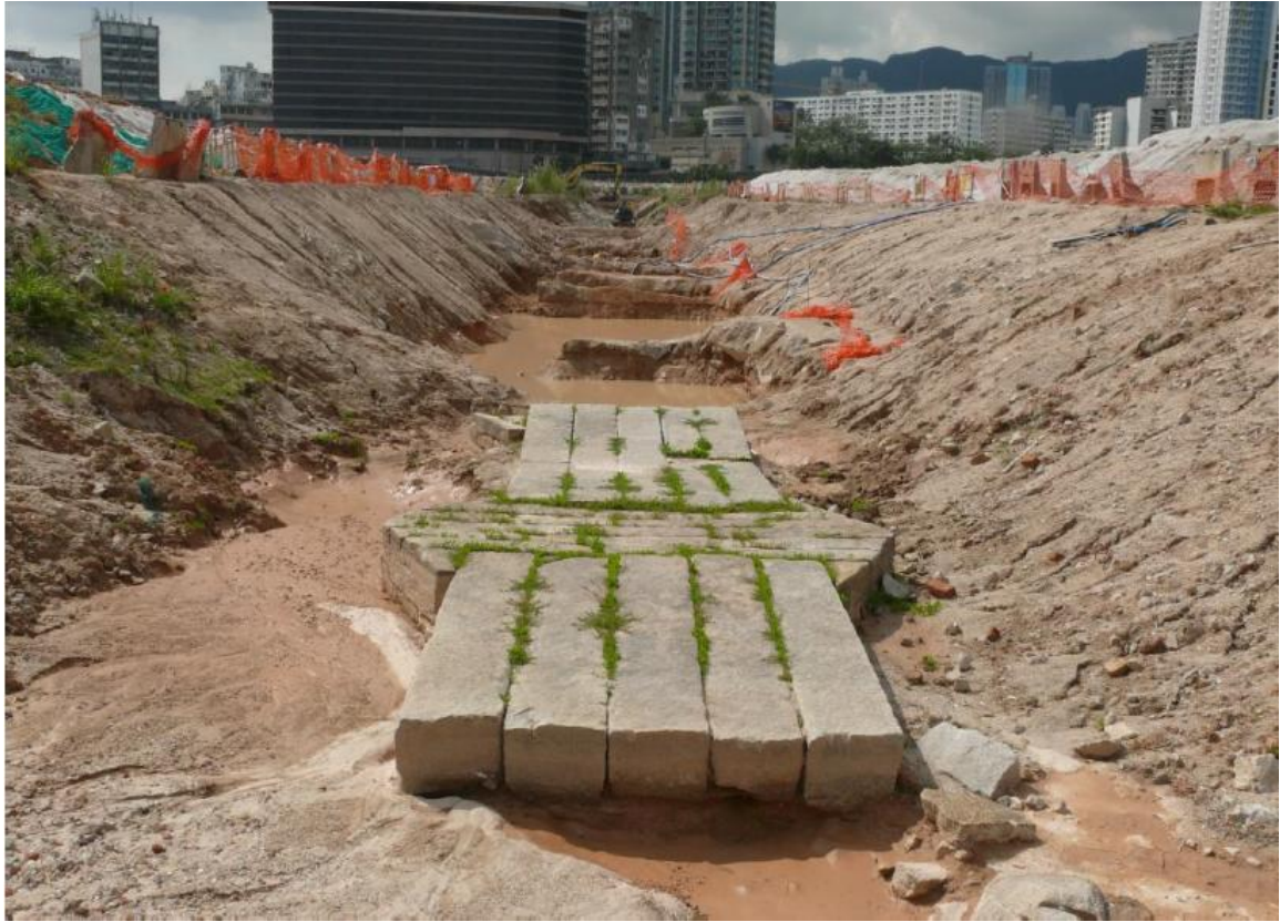
Figure 1-2 North Facing of the Excavation Site
