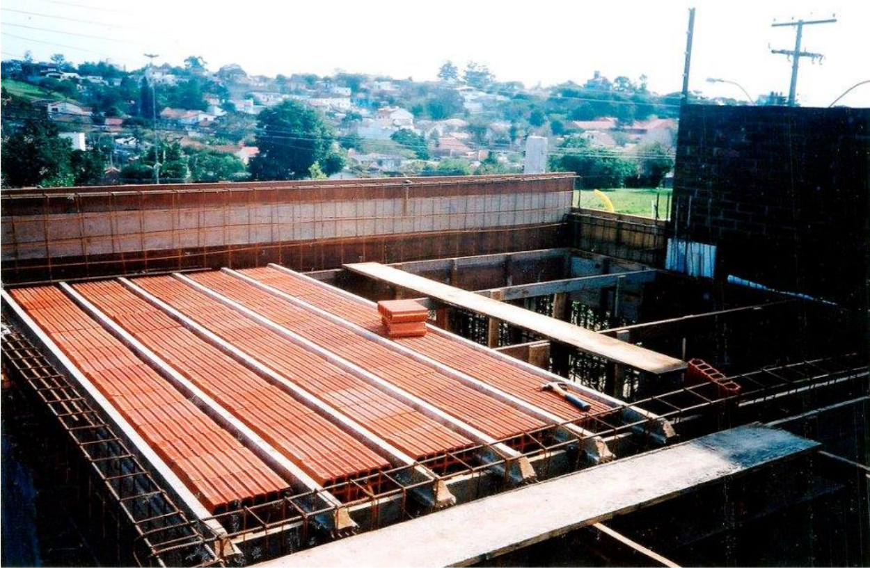
Figure 3-17 – Installation of prefabricated slab system [18]
