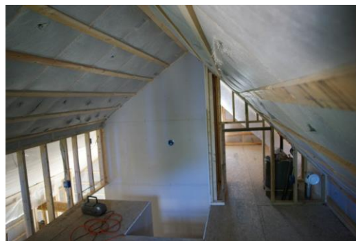
Figure 3-23 - Cellulose Batt Panel [15]
