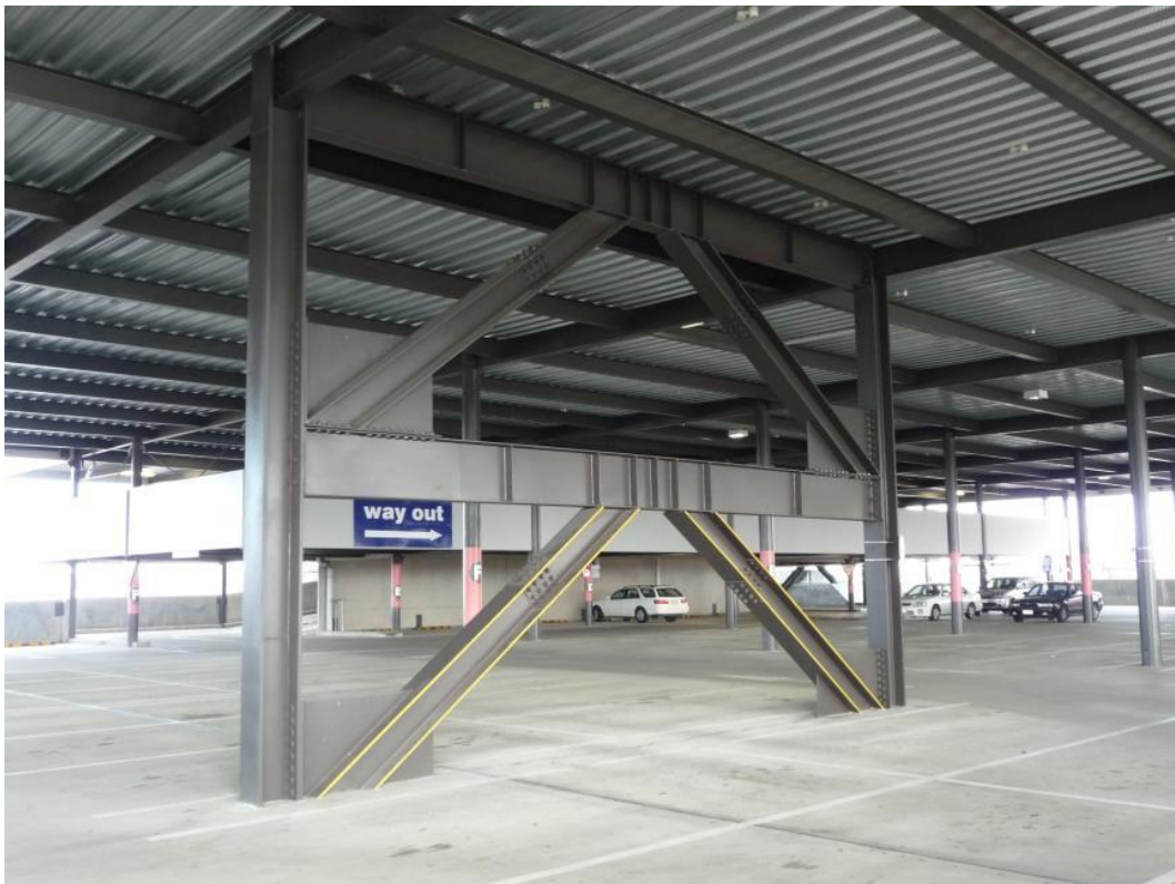
Figure 23: Eccentrically braced frame example
