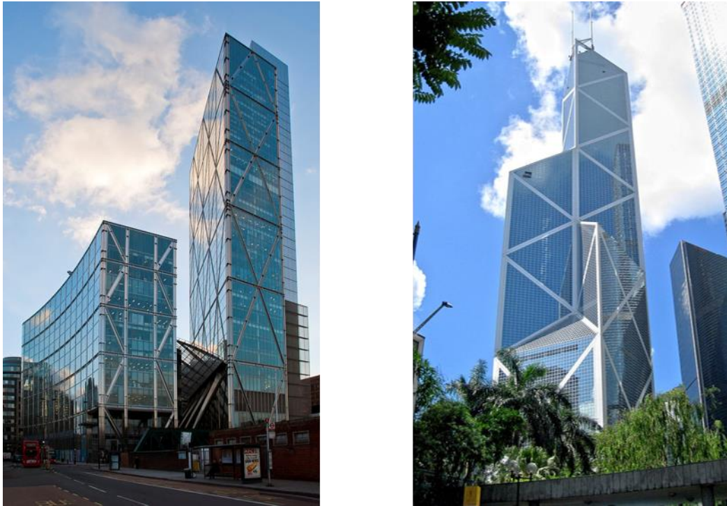
Figure 9: Broadgate Exchange House in London, UK; Bank of China Tower in Hong Kong
