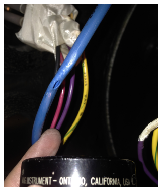
Figure 5.61: Anode gas line melted under irradiated heat flux.
