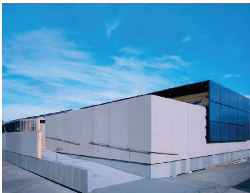
Fig.9.2.12-MED in Italy, vista esterna
