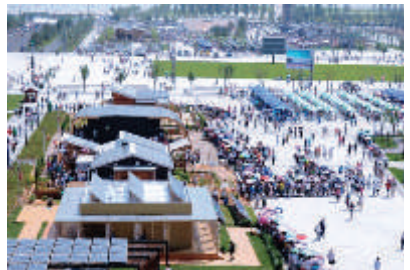
Fig.1.2.7 -Solar Village Beijing 2013
