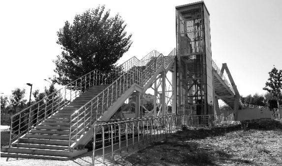
Figure 49. Pedestrian overpass (personal archive, 2014)
