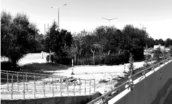
Figure 50. Pedestrian overpass (personal archive, 2014)
