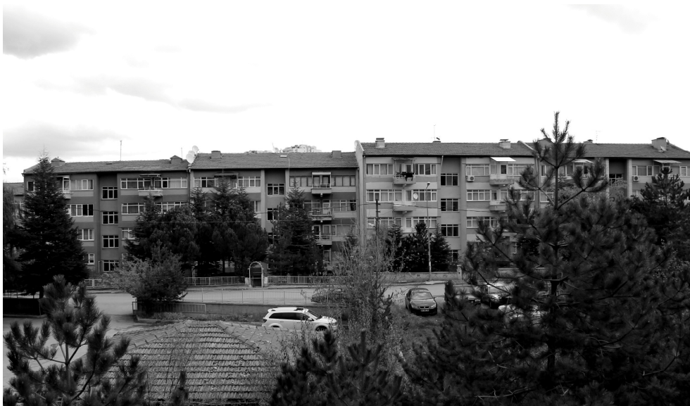
Figure 26. View of 5 storey apartment blocks (personal archive, 2014).
