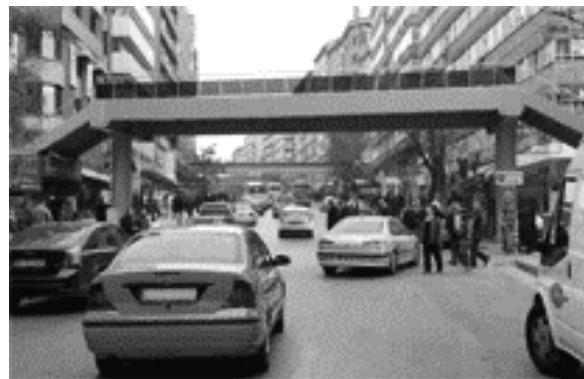
Figure 12. Overpass in city center (Oncu, 2009)
