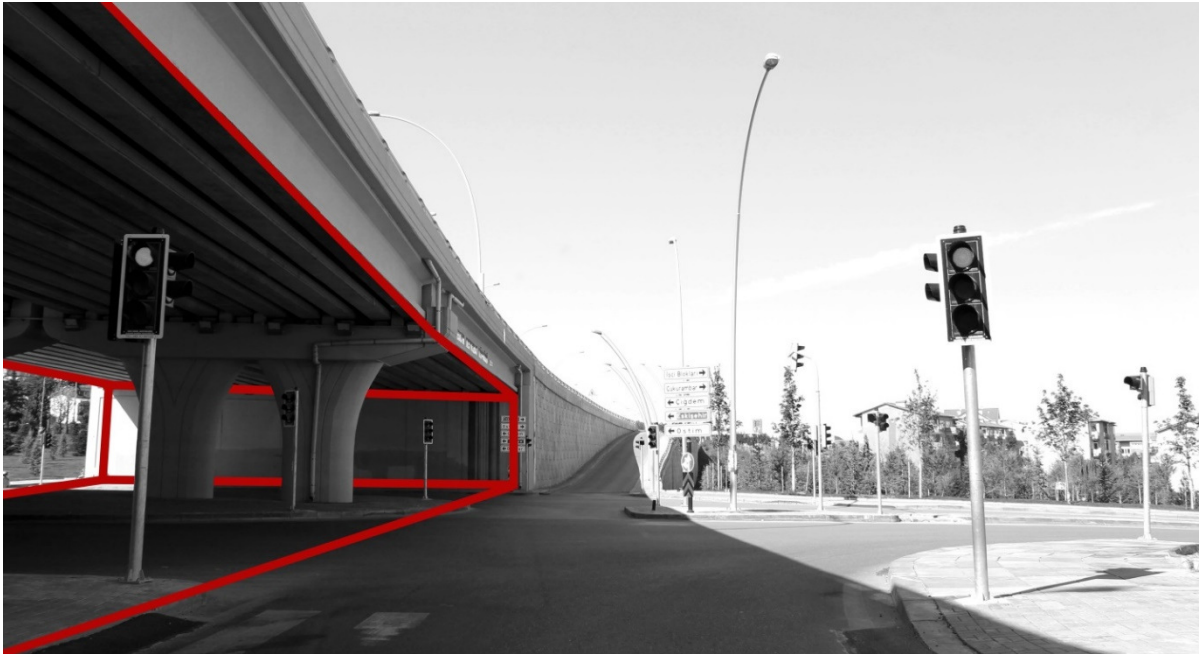
Figure 48. Underpass located at the area (personal archive, 2014)
