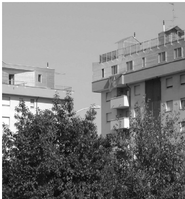
Rooftop housing Albori Cinisello Balsamo 2007
