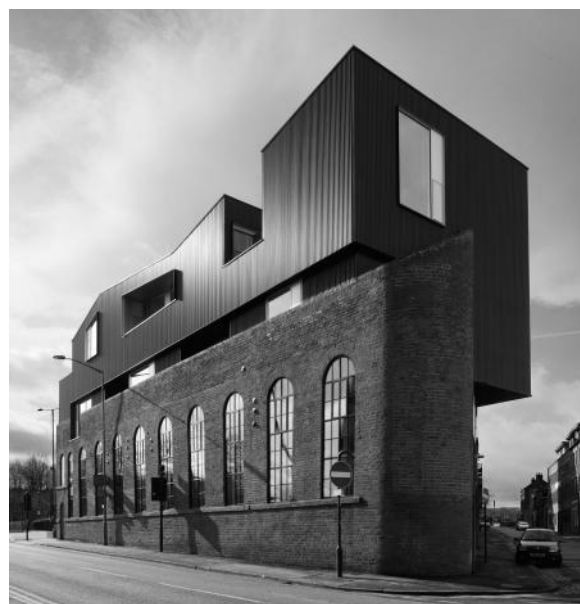
Shoreham Street office Project Orange Shoreham, UK 2012
